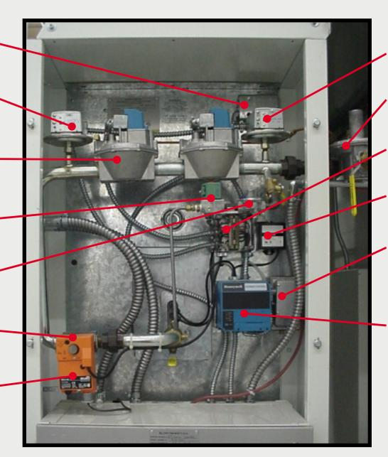
LOW PRESSURE SWITCH Honeywell C645A1030
